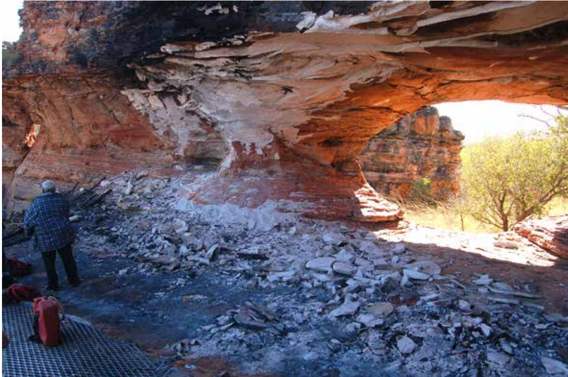
Figure 8. Fire damage has resulted in the loss of valuable paintings. The shattered sandstone on the floor of the shelter was considered unsalvageable.
