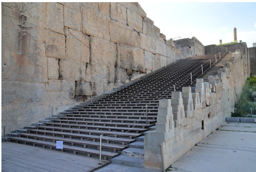
Figure 1. The double stairway to the terrace, cut and fitted from the same mortarless limestone as the platform it ascends.
