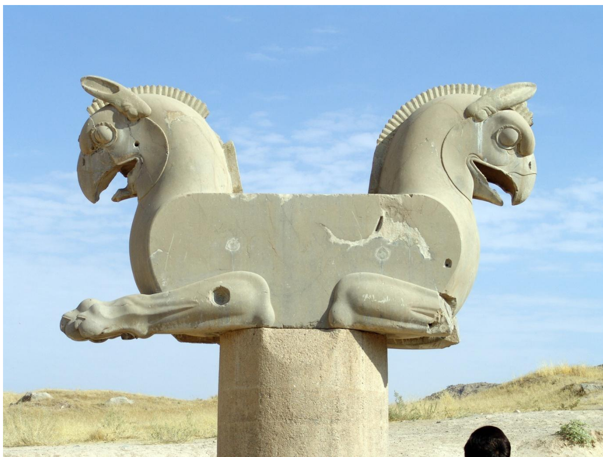
Figure 8. A double-griffin capital from Persepolis, locally called a homa . The upturned ears carried the timber ceiling-beams; the form is structural before it is symbolic.
