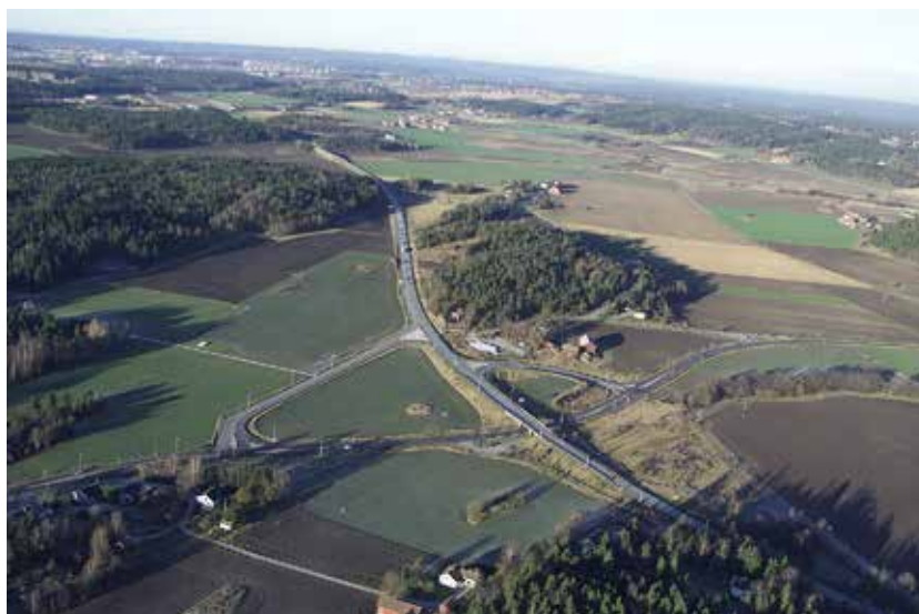
Figure 2. Aerial view of the southernmost part of the research area, before the completion of the new highway. The rock art sites are located on rock exposures close to the road. Photograph: The Norwegian Public Roads Administration.
