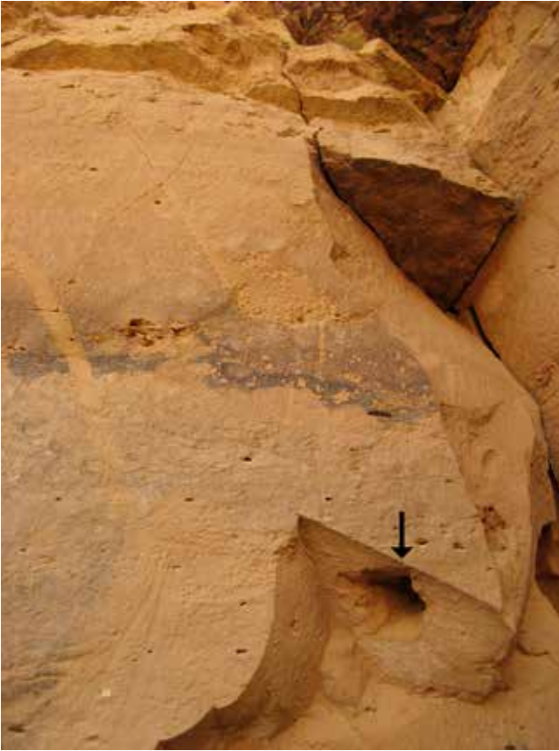
Figure 13. Detail of eyelet, damaged 'giraffe'.
