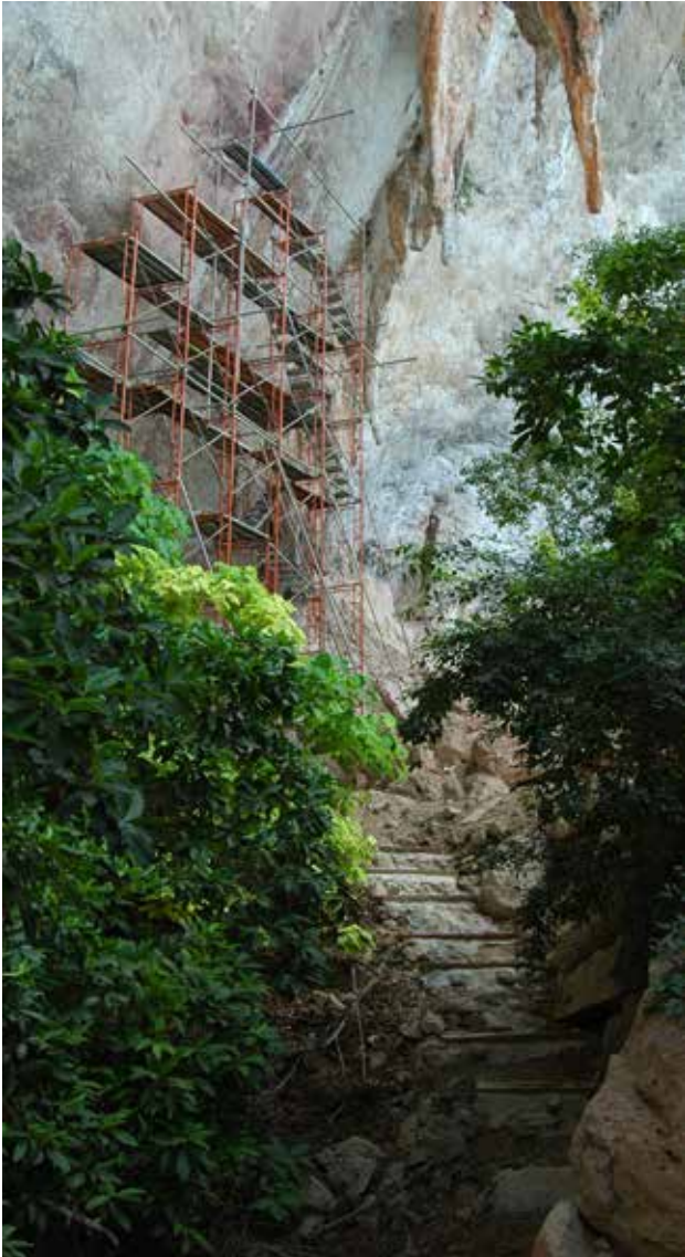
Figure 3. Fieldwork in January 2009. A large scaffold was erected in front of Panel C to provide close-up access to the rock art.
