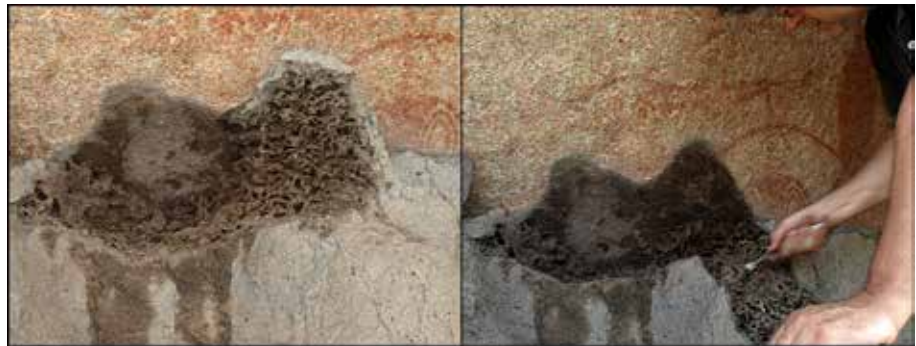
Figure 10. Removal of the inner 50 mm protective buffer zone with small hand tools down to the thin layer of attachment carton (see also Fig. 9, left picture).
