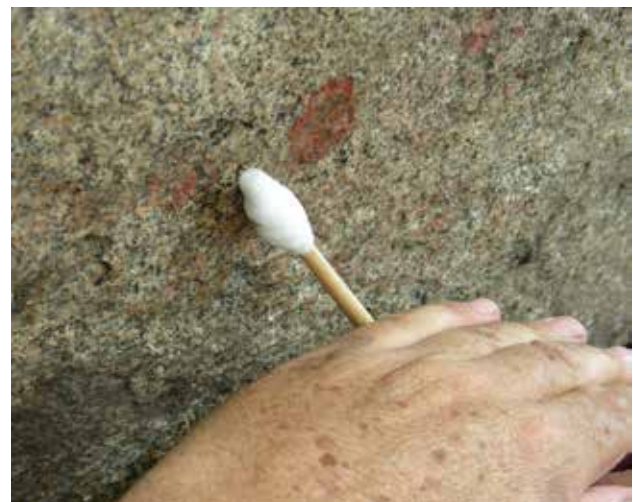
Figure 7. 'Rolling poultice' or moist swab technique.
