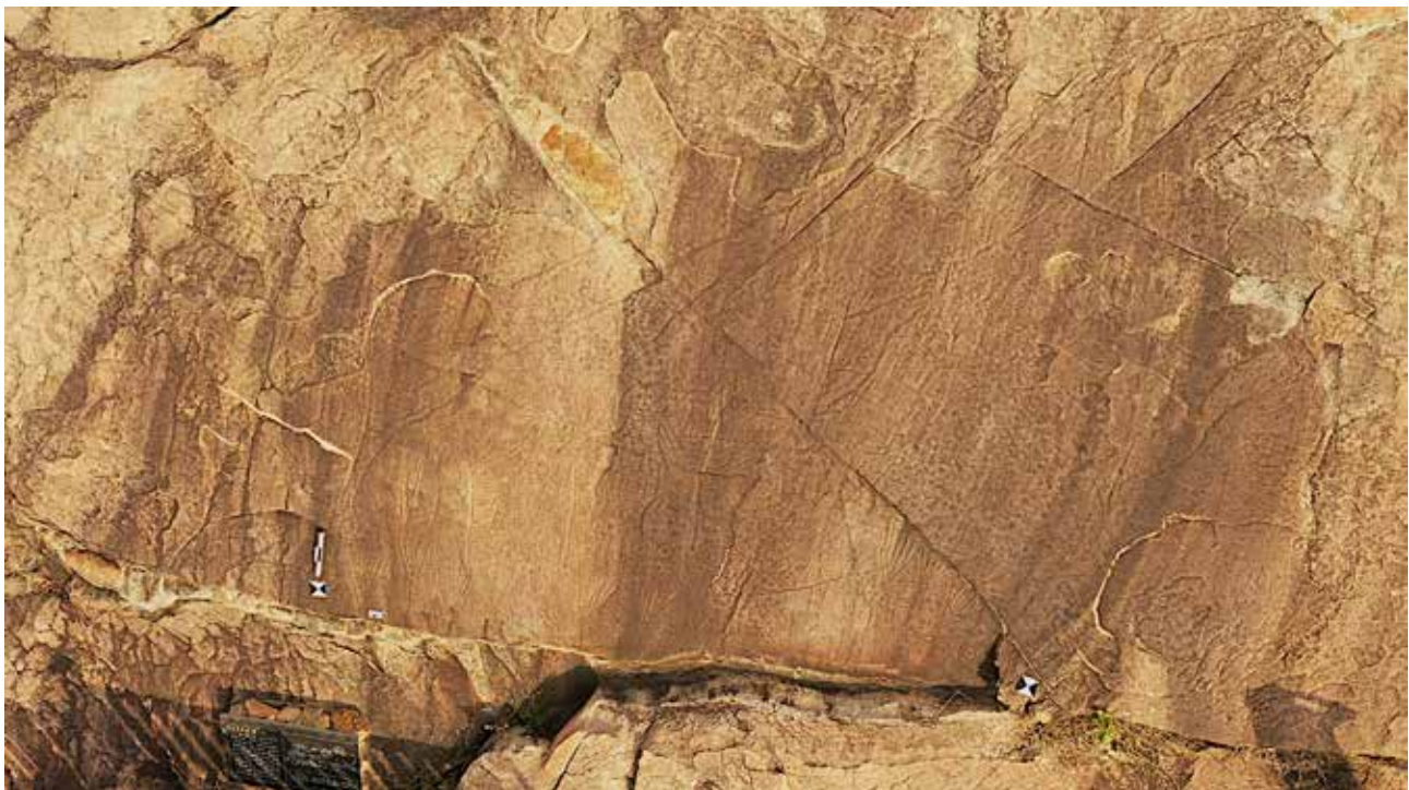
Figure 1. Jiangjunya rock art (see the multiple cracks and traces of reinforcement on the surface). Photo taken in October 2022 by YJ.
