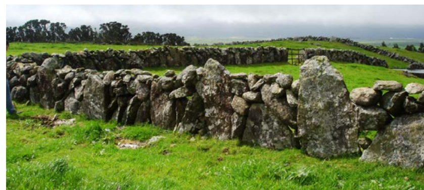
Figure 3. The 'dry stone' walls show the larger stones enclosed in smaller ones (photo TA).
